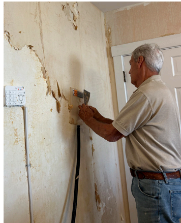
▲ Joe Palfini painstakingly removes old wallpaper, in preparation for a fresh coat of paint.
